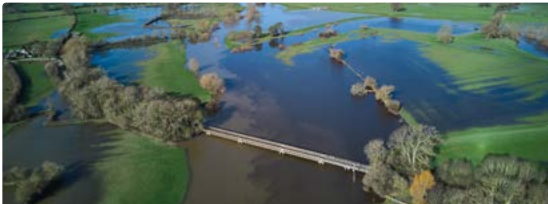
Flooding on the River Severn
